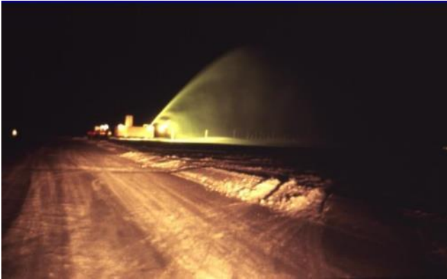
Photo 3: Constructing the Mars spray ice island (January 1986)
