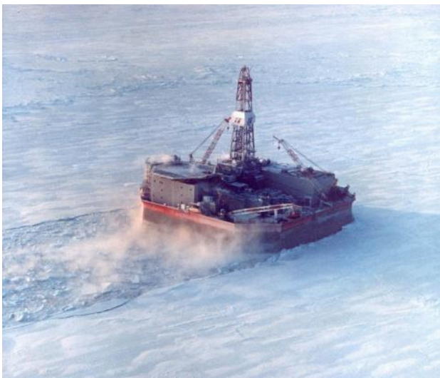
Photo 5: Gulf's Mobile Arctic Caisson (MAC) deployed in the Beaufort Sea
